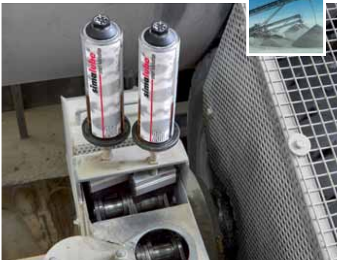
Two 250 ml simalube lubricators with brushes lubricate and clean the chain drive of a drum washing machine.
